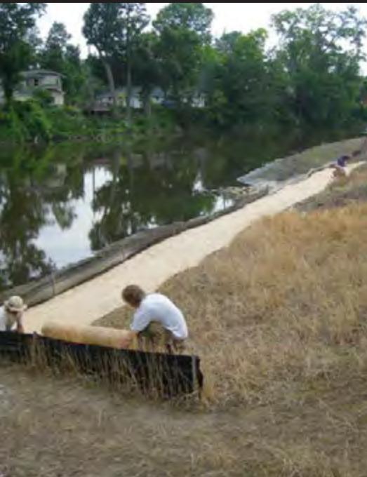
Installation of erosion blanket
