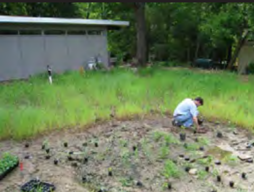
Rain garden planting
